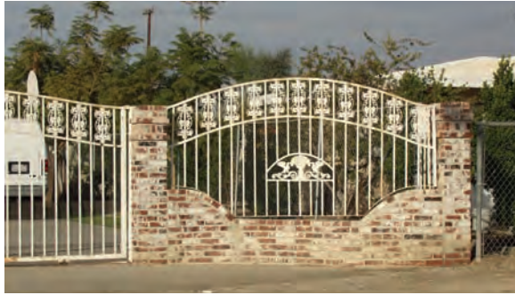
Exhibit 14 | Existing Wrought-Iron Fence
