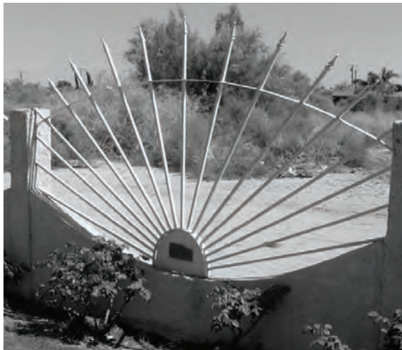
Exhibit 7 | Arch Wall at Catholic Church
