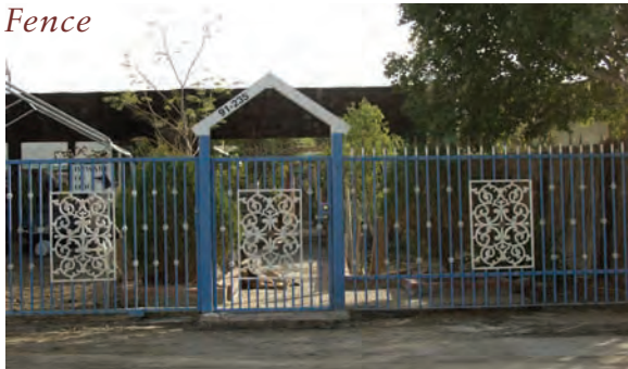
Exhibit 15 | Existing Wrought-Iron Fence
